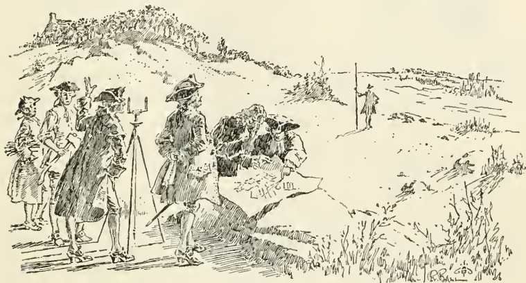
SURVEYORS LAYING OUT BALTIMORE
